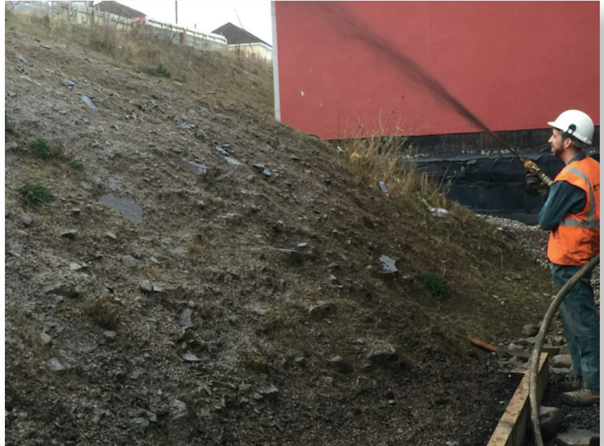
Biotic Earth applied over existing conditions where previous seeding operations failed.
