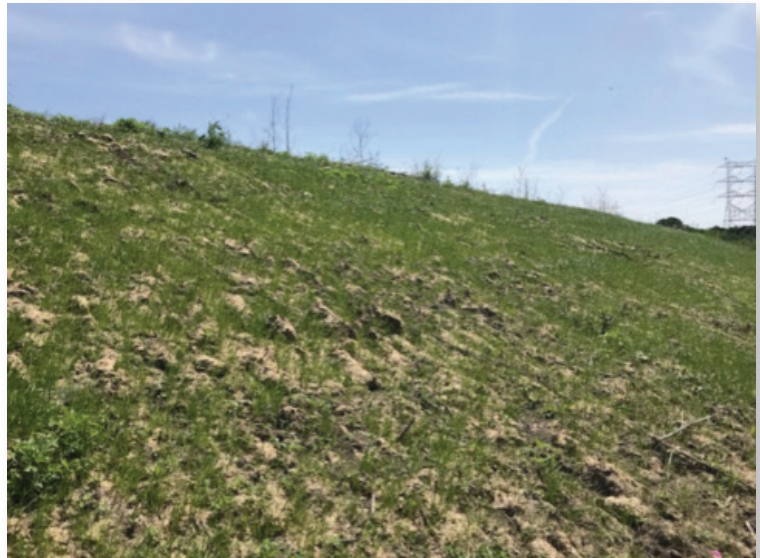
Significant vegetation achieved within one month of installation: April, 2018.
