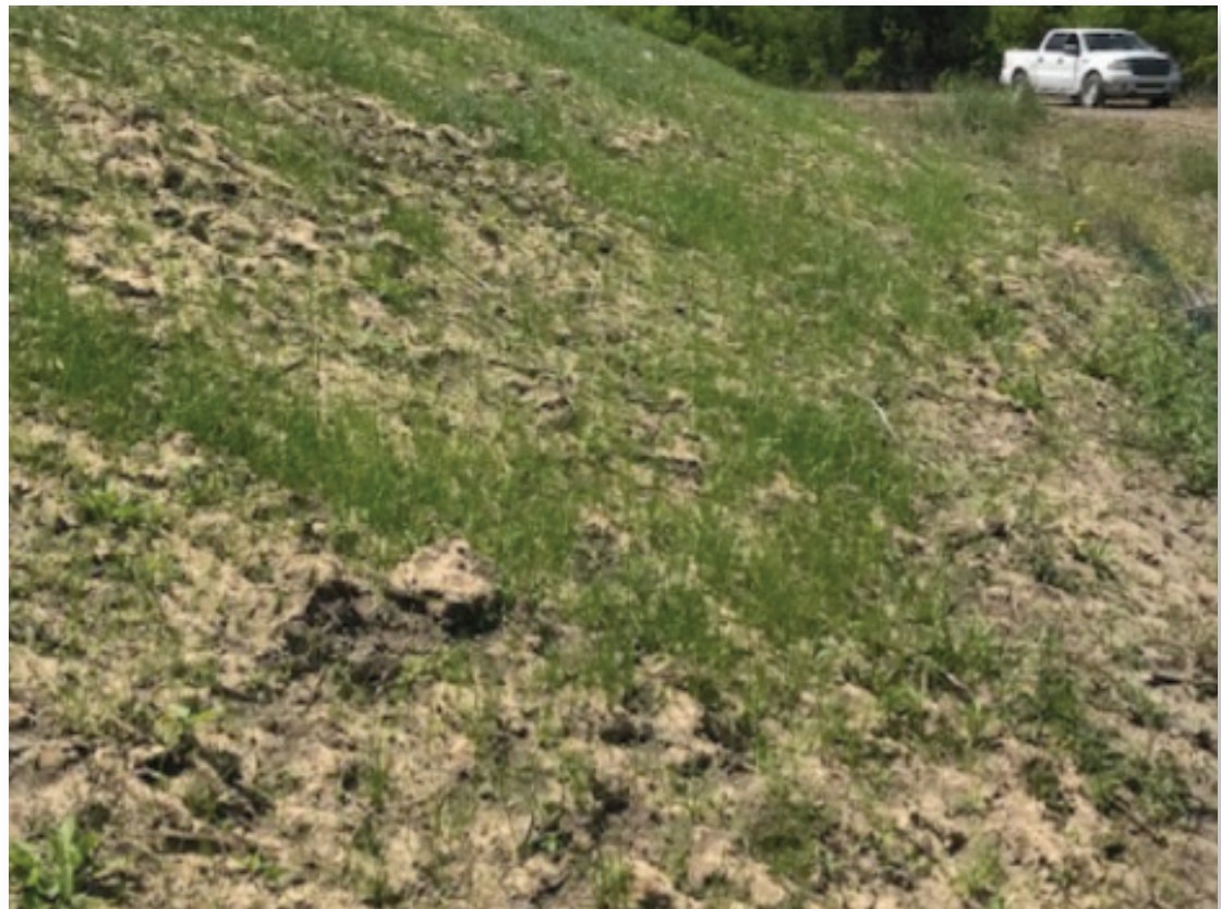
One month post installation .
